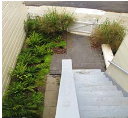
Completed L2L Installation.
