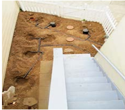
L2L tubing and mulch shields in place.
