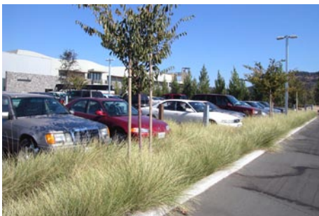
Example of a Parking Lot with Bioswales
