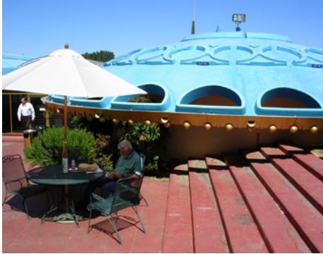
Courtyard at south end of Administration Building
