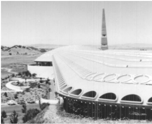
Marin Civic Center Roof and Spire - 1970
