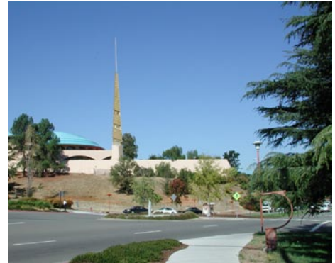
Civic Center Drive
