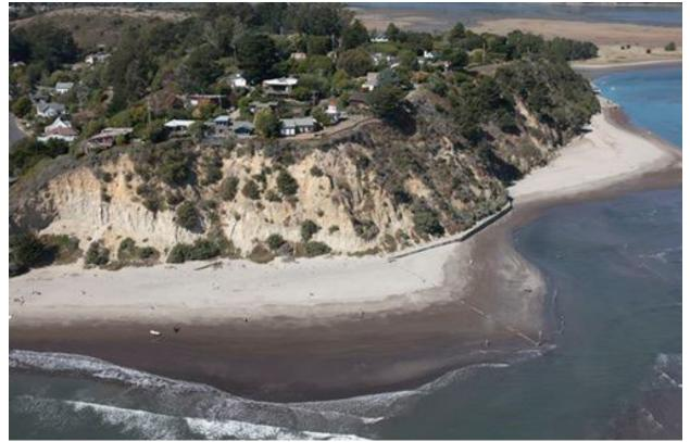
Shoreline armoring like this seawall leads to loss of sand generating materials and a loss of beach, effectively leading to ocean/bay waters covering such beaches at all times as sea levels rise. In contrast, where natural erosional processes are allowed to continue, beaches themselves can adapt and reform. This slide shows both circumstances
