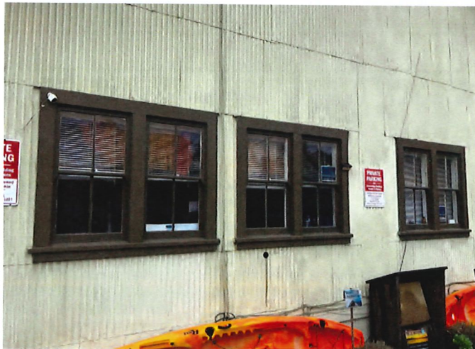
Historic window fabric and placement, January 21, 2024.
