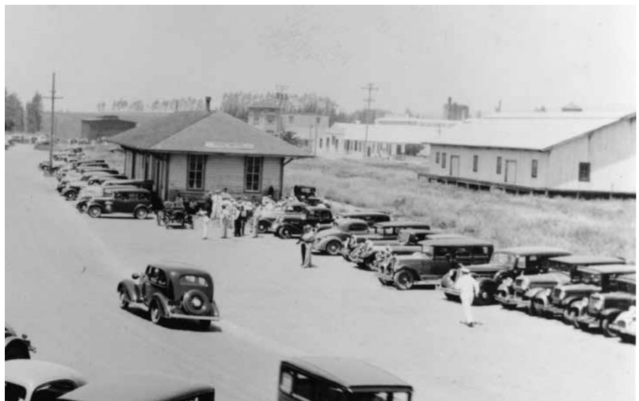
At far right, Leland S. Murphy's "pea shed" in situ in the former railyards of Point Reyes Station, 1930s. Jack Mason Museum of West Marin History.
