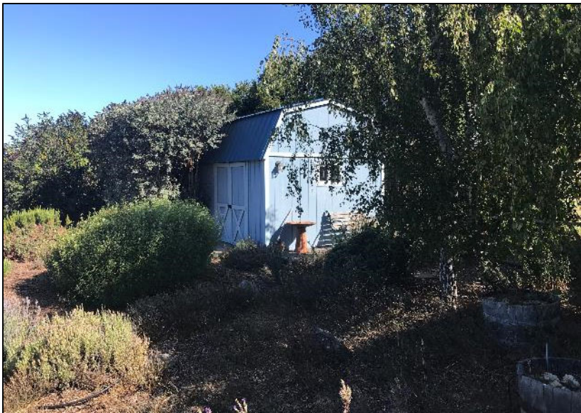
Outbuilding in the northwestern portion of the developed area
