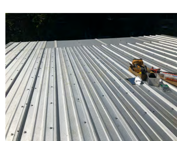
1 RIBBED GALVALUME STEEL ROOF
