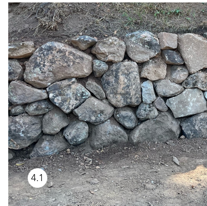
4.1 STACKED STONE RETAINING WALLS
