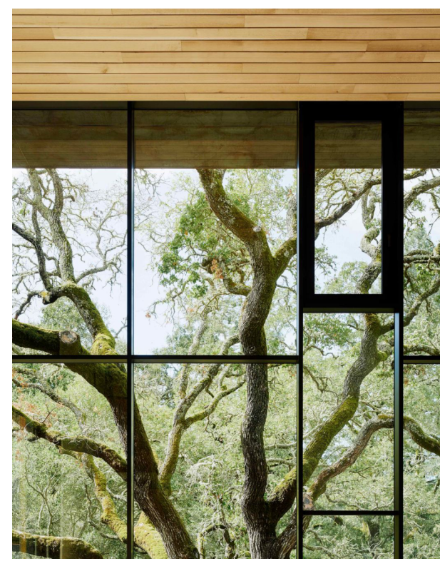
4 BRONZE ANODIZED ALUMINUM MULLIONS AND CLEAR GLAZING
