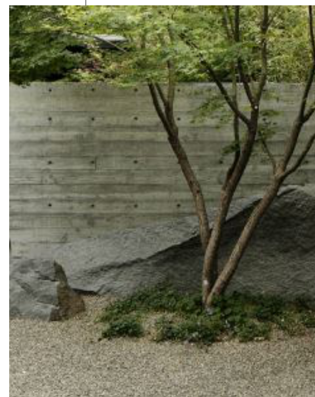
7 BOARD FORMED CONCRETE
