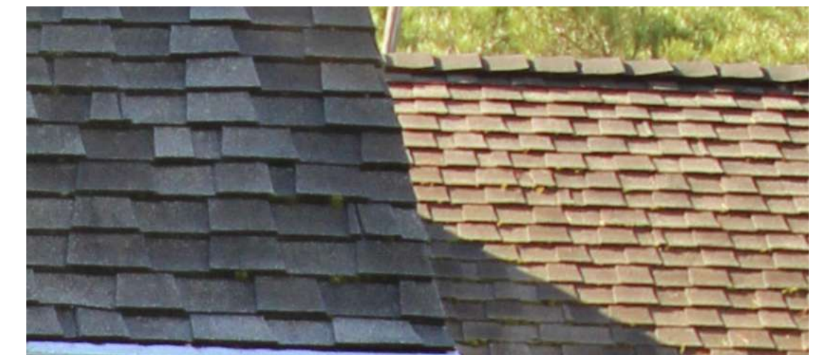
Existing Asphalt Shingle Roof to Remain
