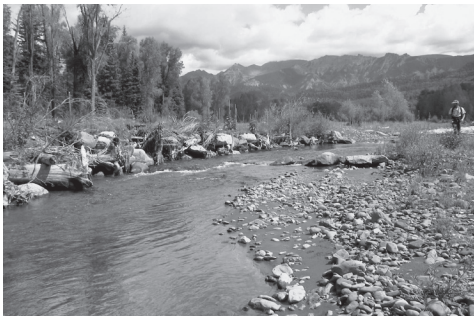
Large woody debris bank protection. Repair by Wildland Hydrology.
