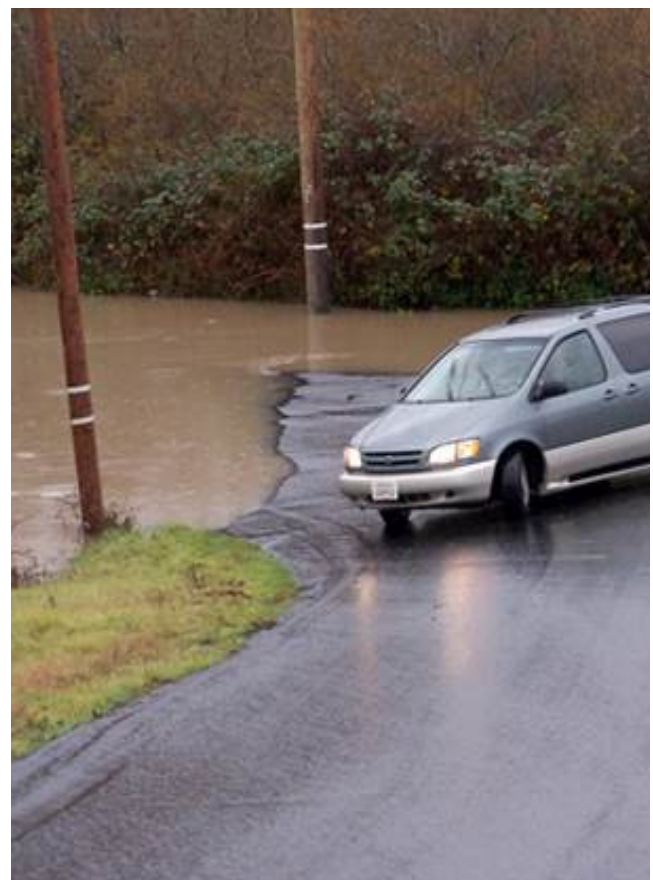
Flooded roads block access Est. date, 1990's. Credit: CDA
