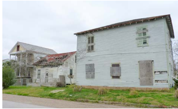
Galveston, Texas home before elevation. Credit: Galveston Historical Foundation
