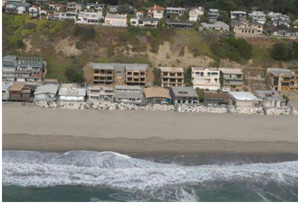
Bunker-style coastal homes in Santa Cruz feature elevated ground floors intentionally allowed to flood.
