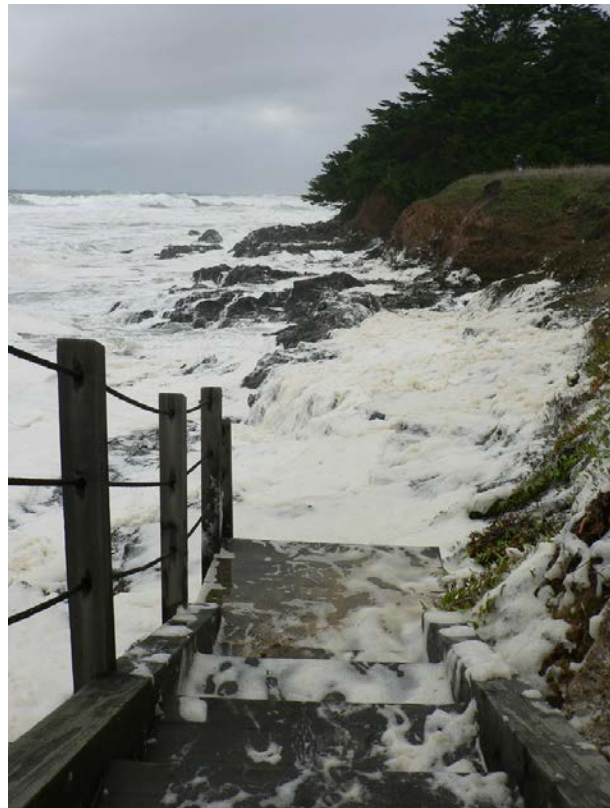
Bolinas public stairwell flooding, 2013. Credit: A. Rappaport
