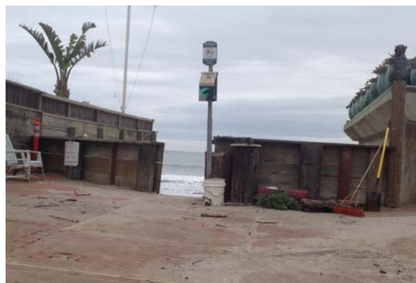
Gaps between buildings and walls such as this one at Stinson Beach represent possible floodgate locations.
