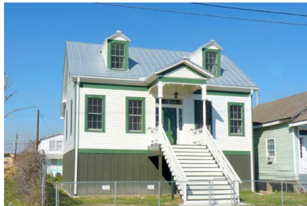
Continuous foundation wall. Credit: Galveston Historical Foundation
