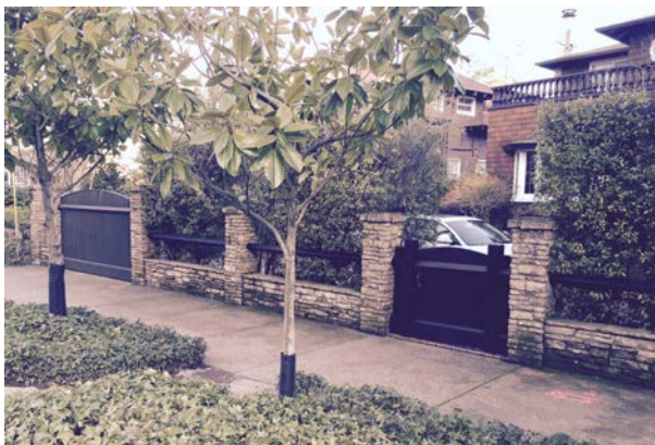
Flood wall and gate in masked with landscaping. Credit: E. Doldan Schujman
