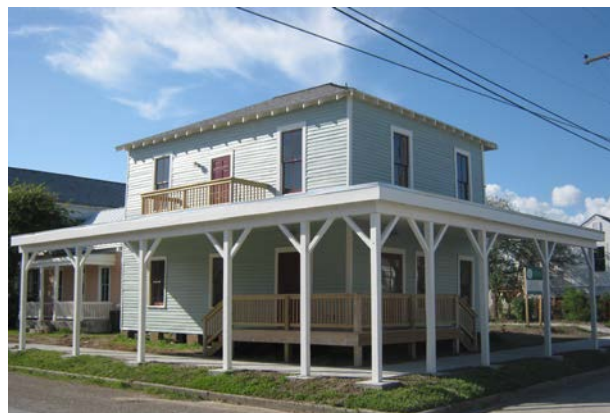
Galveston, Texas home after elevation. Credit: Galveston Historical Foundation
