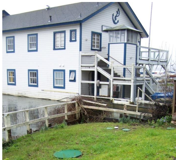
Inverness Yacht Club septic system covers. Credit: S. Callow
