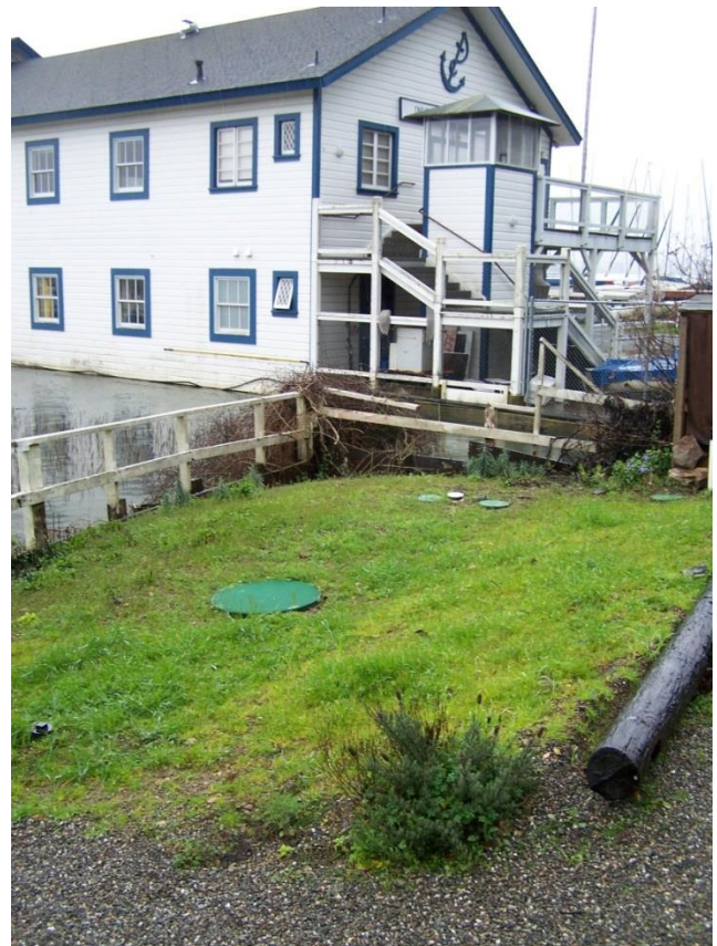
Inverness Yacht Club septic system covers. Credit: S. Callow
