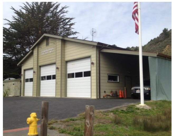
Stinson Beach Fire Station No. 2 is vulnerable. Credit: CDA
