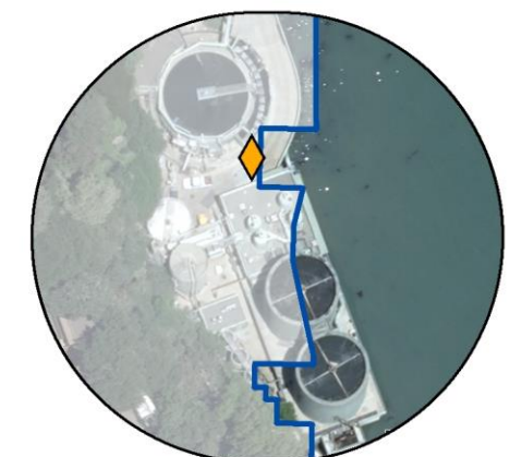
4: Sausalito Marin City Wastewater Treatment Plant
