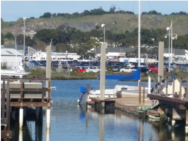
View of Larkspur Ferry parking lot and boats from Greenbrae Boardwalk. Credit: BVB Consulting LLC
