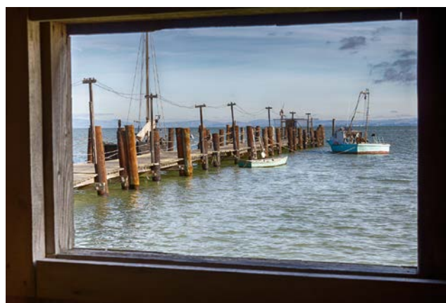
December 12, 2016 king tide floods China Camp historic pier. Credit: R. Rothbart
