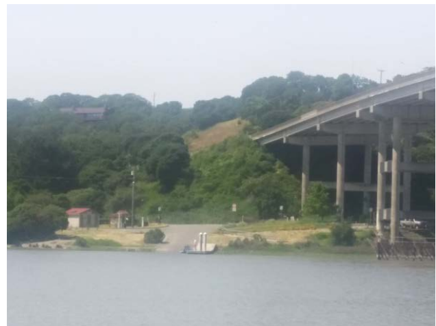
Black Point Boat Launch at State Route 37 and the Petaluma River. Credit: BVB Consulting LLC
