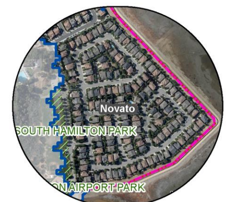
6: Lower Hamilton Levee
