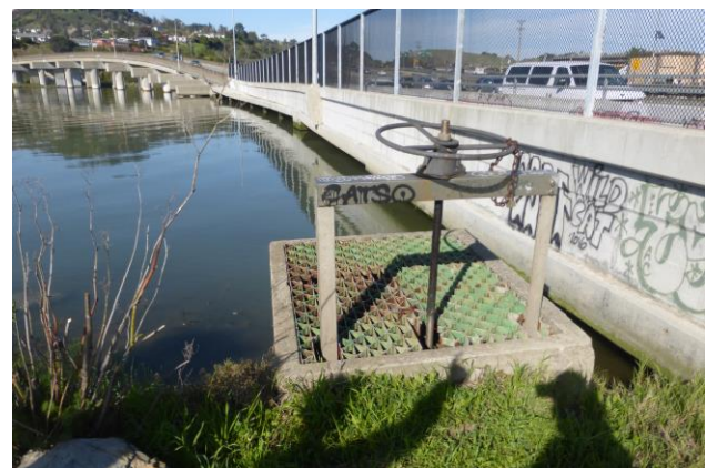
Corte Madera Creek at the end of Lucky Drive. Note the low-lying segment of US Highway 101 starts here. Credit. Marin County DPW
