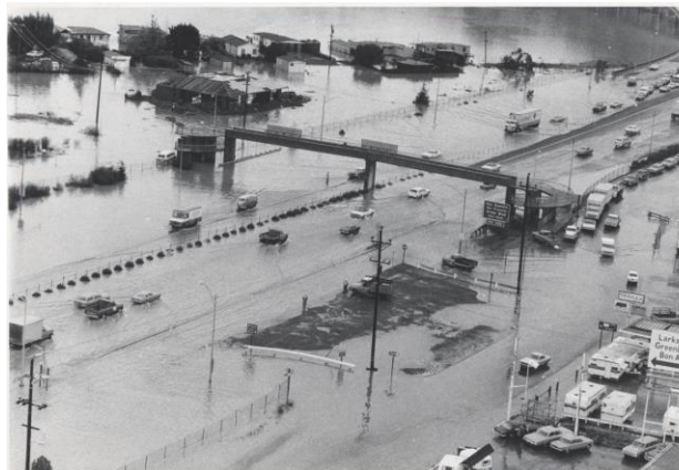
1973 Flood on US Highway 101 and fronting marshes. Larkspur. Credit: Marin County DPW
