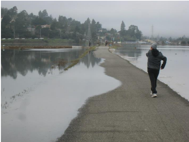
Mill Valley/Sausalito Multi-modal Pathway. Dec. 2014 King Tides. Credit: DPW
