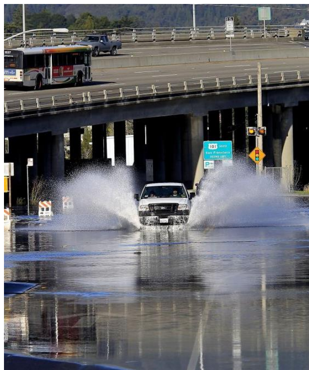
US Highway 101 on ramp at Manzanita is already flooded at high tides, especially combined with storms. Credit: Unknown
