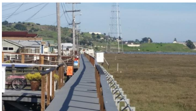
Greenbrae Boardwalk. April 2016. Credit: BYB Consulting LLC
