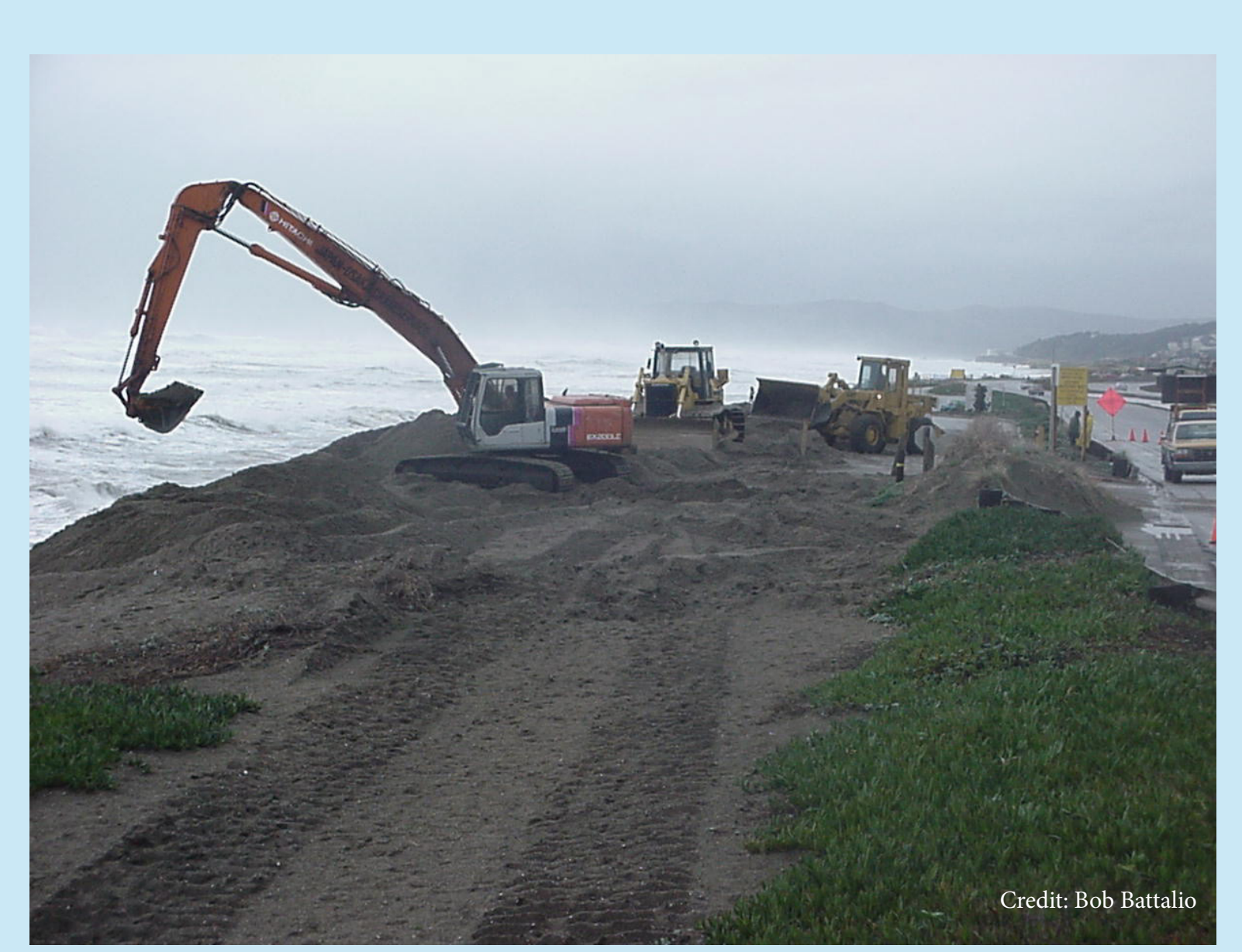
Sand embankment construction for sacrificial erosion projection
