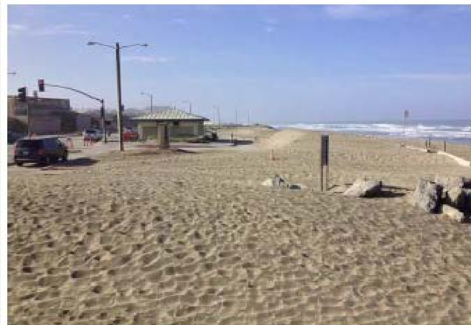
Figure 20 Photos of sand embankment and wind-blown sand transport on April 30, 2013, after the 2012 sand backpass project (© Bob Battalio)
