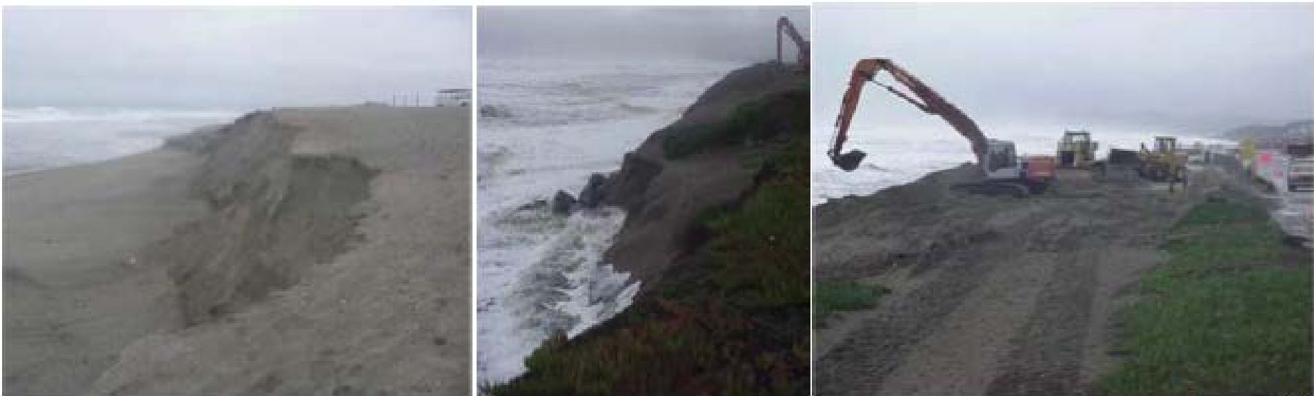
Figure 19 Photographs of Sand Placement in 1999-2000 at Reaches 1 and 2, between the South Parking Lot and the SWOO (© Bob Battalio)
