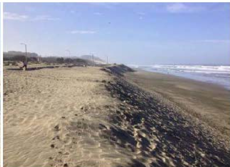
Figure 20 Photos of sand embankment and wind-blown sand transport on April 30, 2013, after the 2012 sand backpass project (© Bob Battalio)
