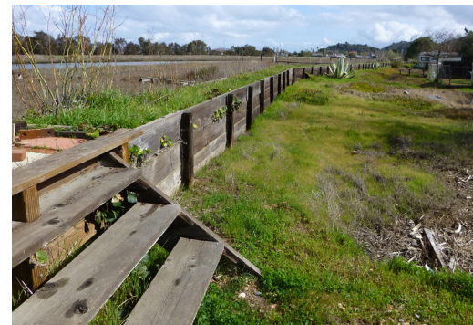
Levee along Gallinas Creek in Santa Venetia Marin County CDA
