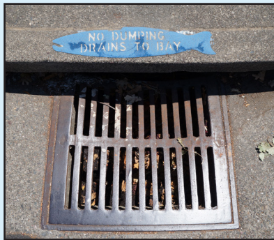
Storm drain on Vendola Drive
