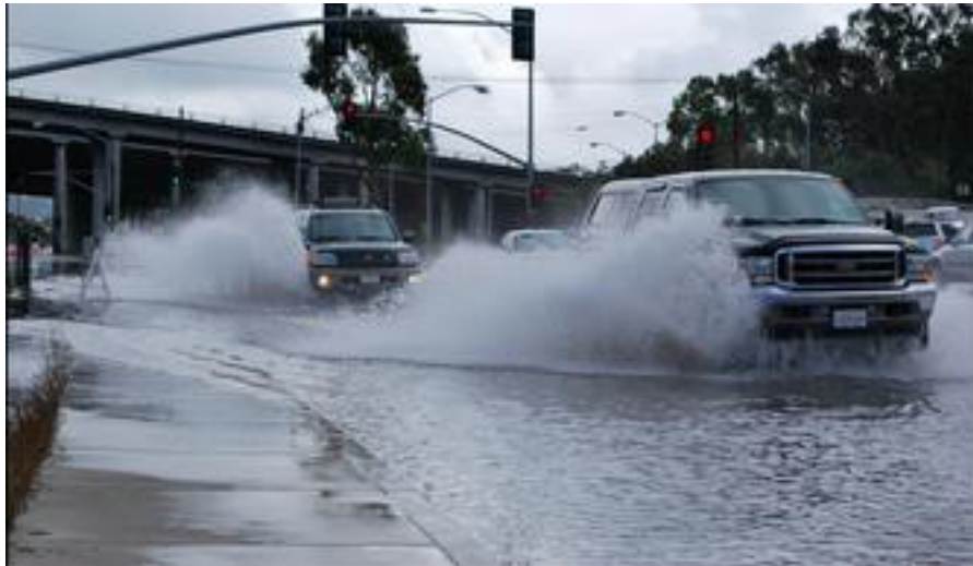
Flooding at Manzanita
