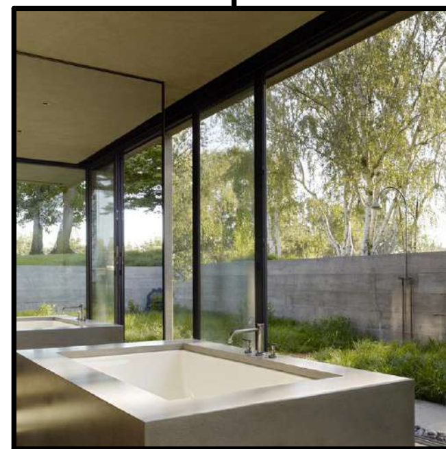
5 WND-1: ALUM. MULLIONS & CLEAR GLAZING COLOR: DARK BRONZE ANODIZED MANUFACTURER: GC FURNISHED
