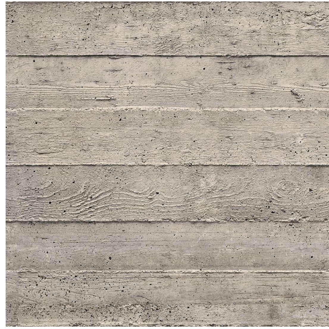
CO-1: BOARD-FORMED ARCHITECTURAL CONCRETE SIMILAR TO (E)
