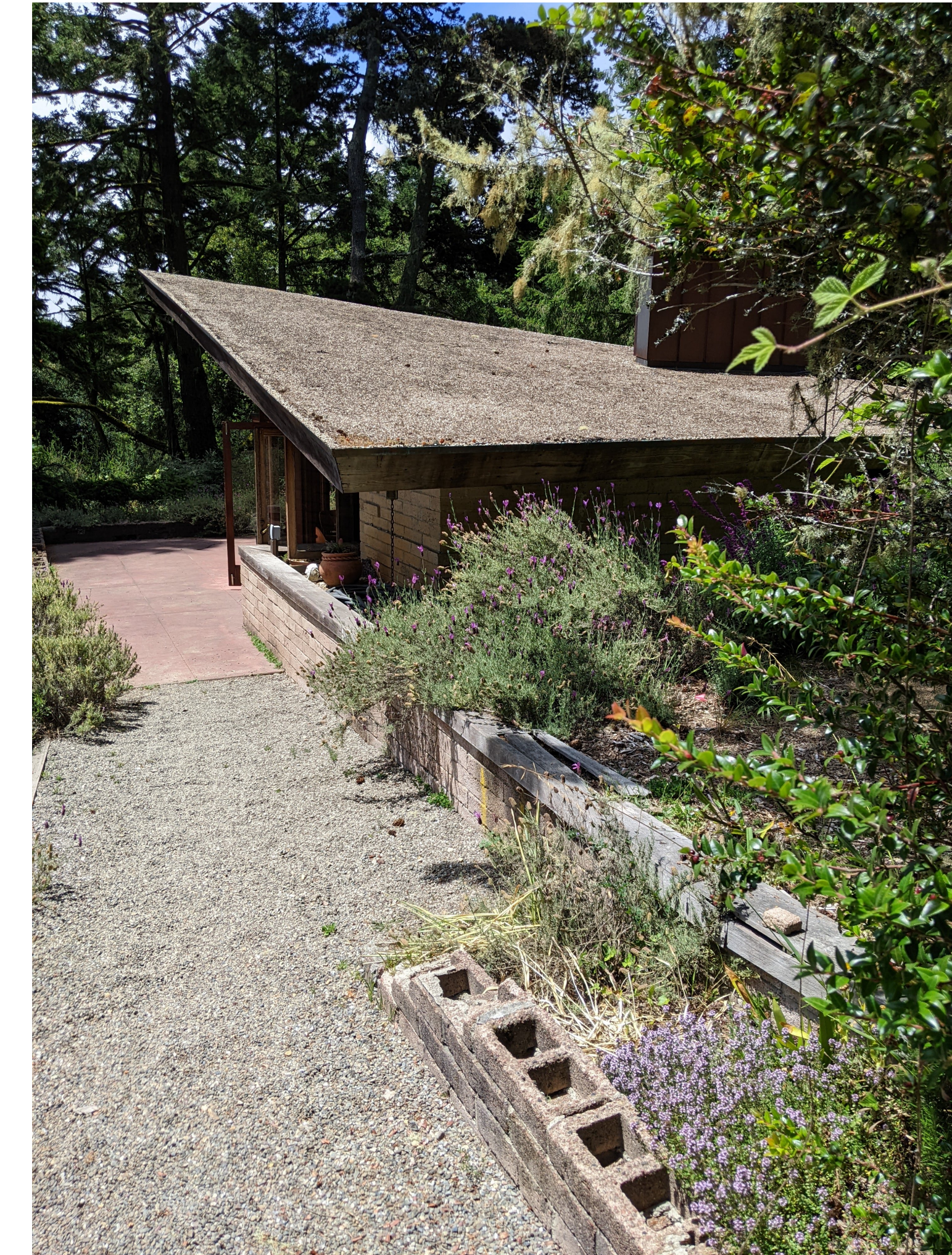
EAST ELEVATION SITE VIEW
