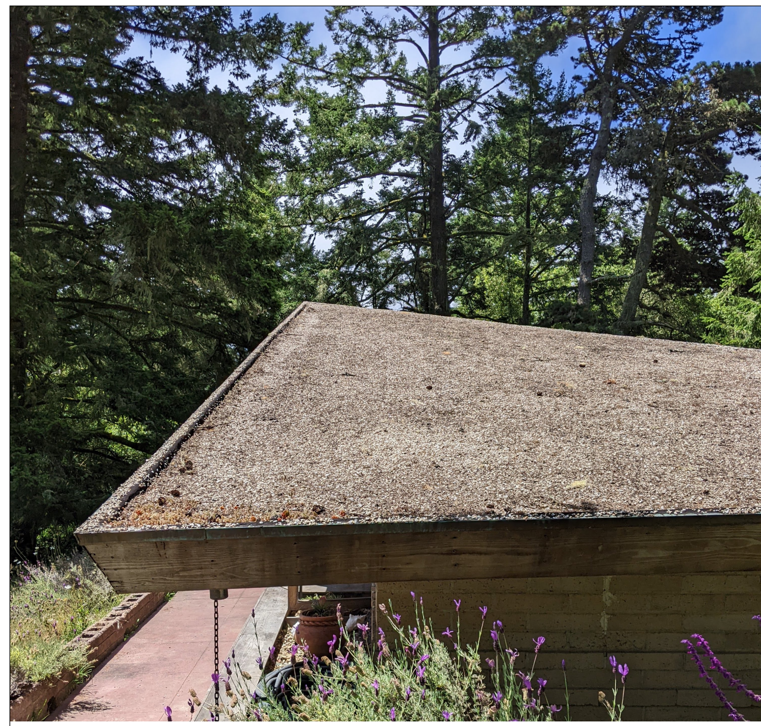
GRAVEL BALLAST TO MATCH ORIGINAL ROOFING MATERIAL
