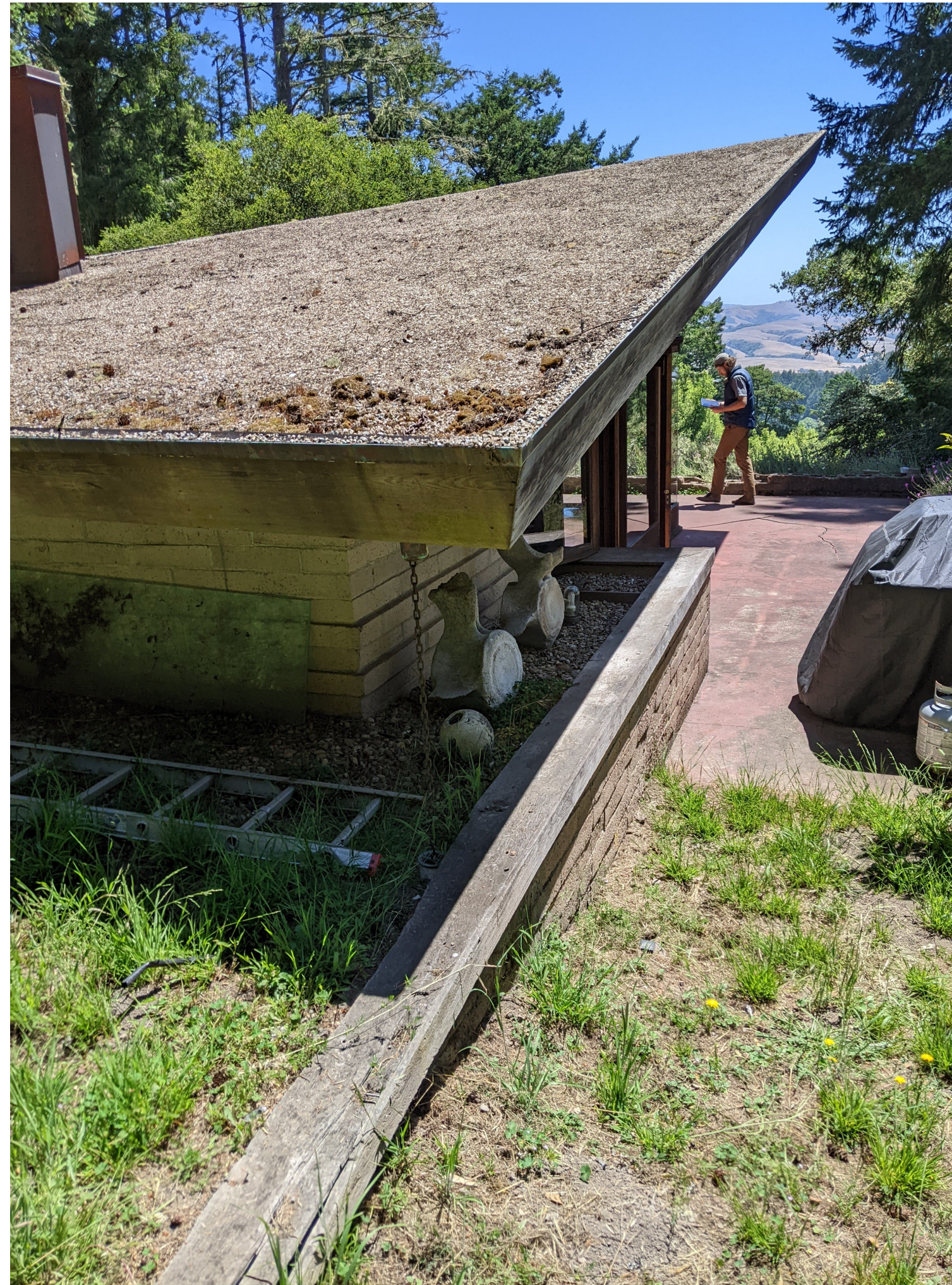
WEST ELEVATION SITE VIEW
