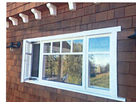
EXISTING WINDOWS & EXTERIOR LIGHTING - ADDITION TO MATCH EXISTING
