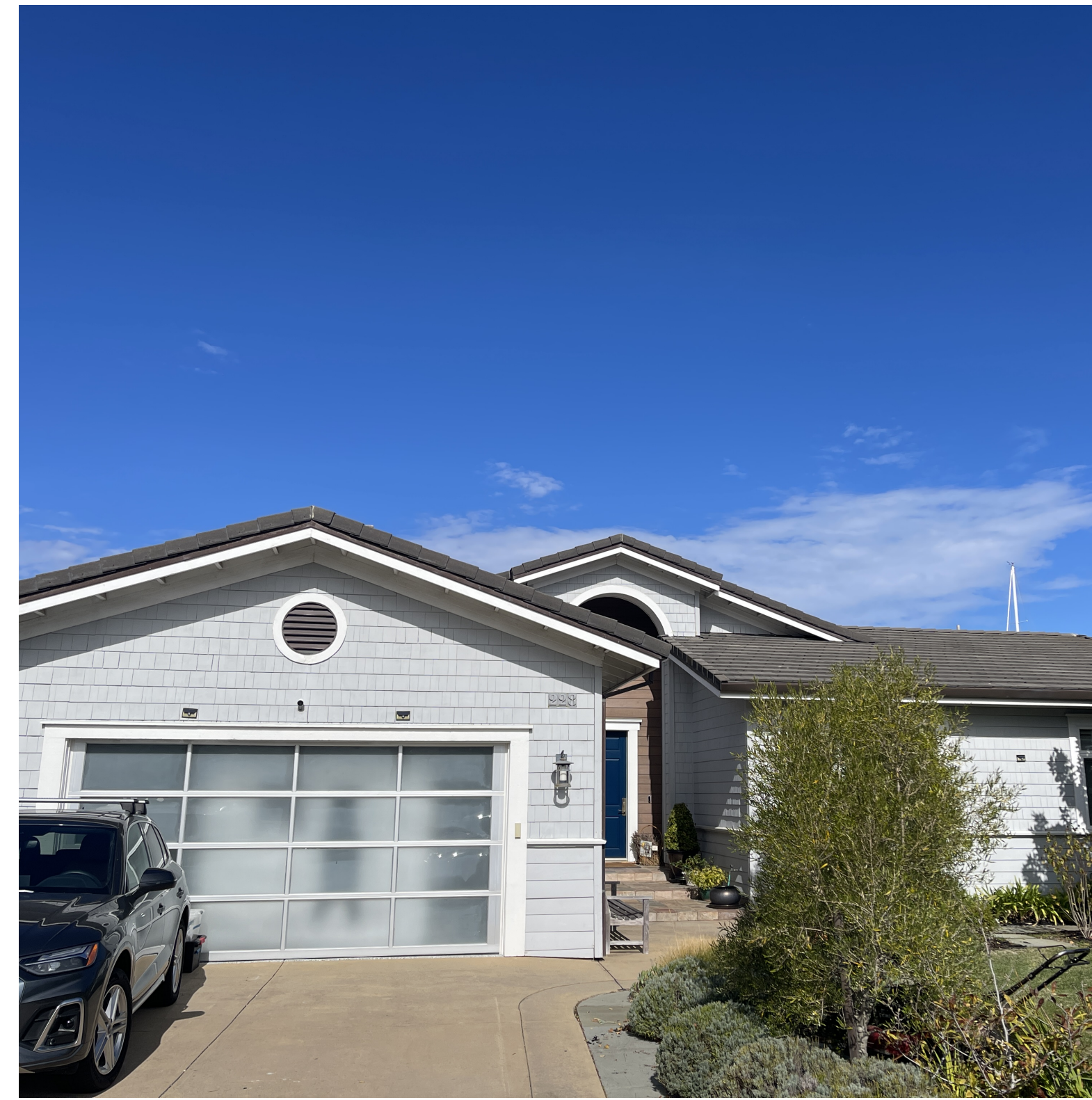
EXISTING ROOFING: CHARCOAL GREY ASPHALT SHINGLES
