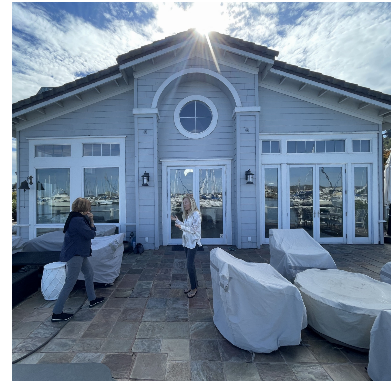
EXISTING WINDOWS: WHITE FRAME EXISTING TRIM: WHITE PAINTED WOOD TRIM
