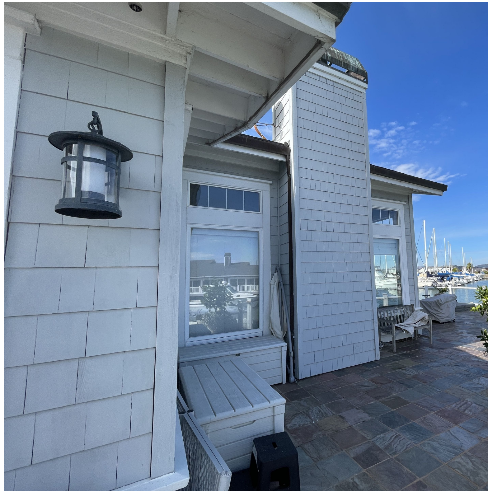
EXISTING SIDING: STRAIGHT EDGE SHINGLE SIDING
