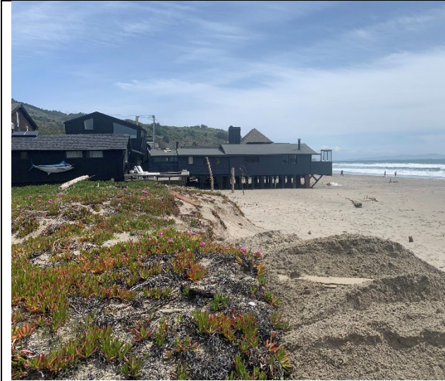
View 2: View of the Project site looking southeast from Upton Beach, April 18, 2023.
