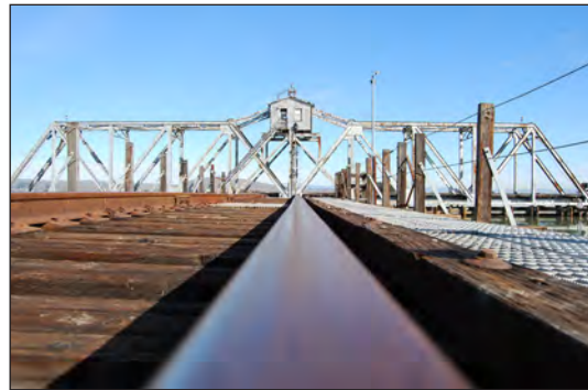
Swing railroad bridge across the Petaluma River Photo credit: Susanna Mahoney
