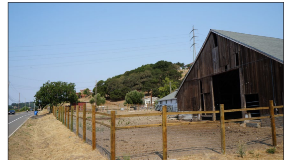
Old barn on Atherton Ave.
