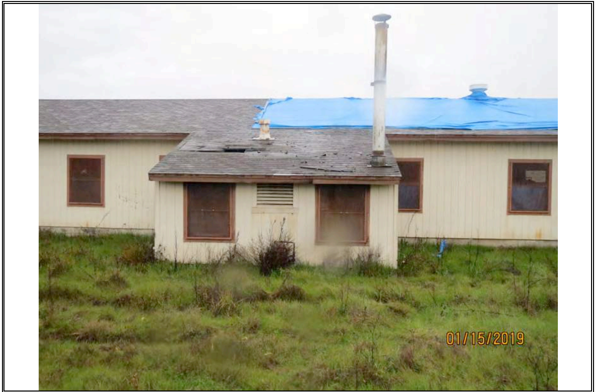
Photograph Number 5: View of the building on the Property (looking north)
