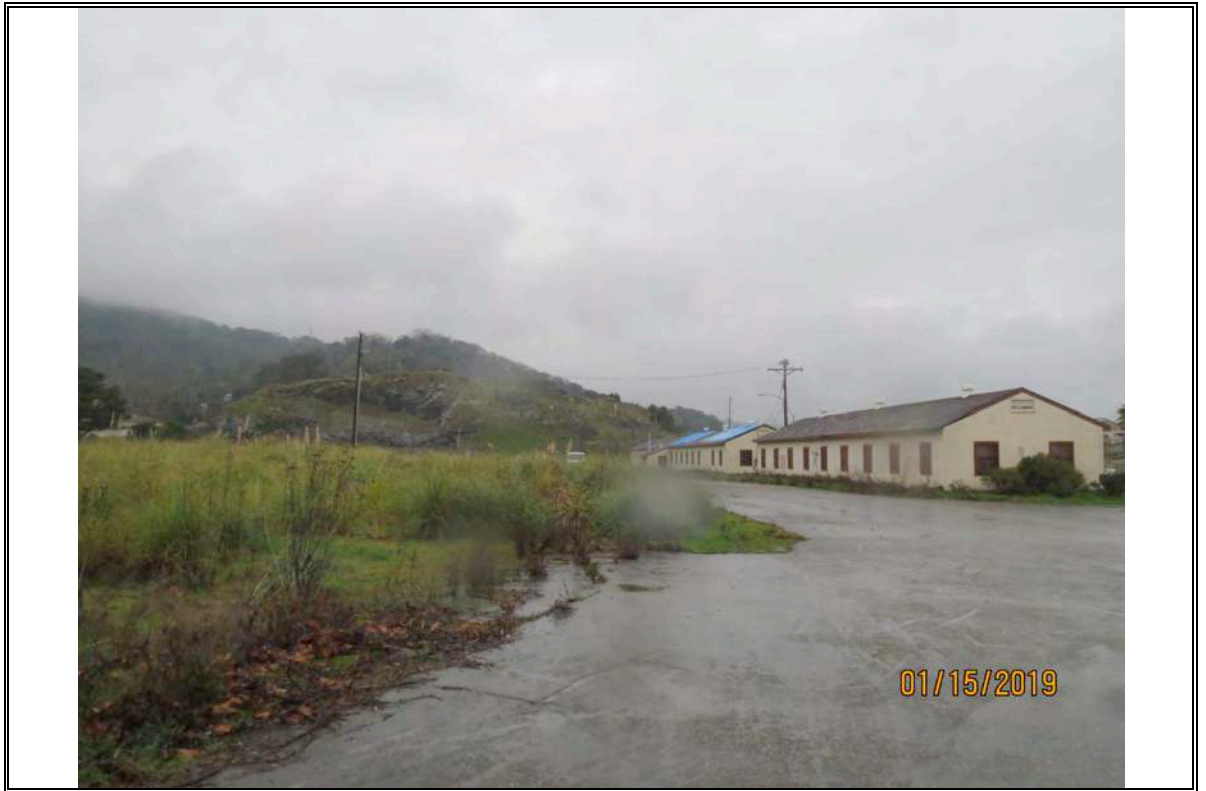
Photograph Number 3: View of the buildings on the Property (looking west)
