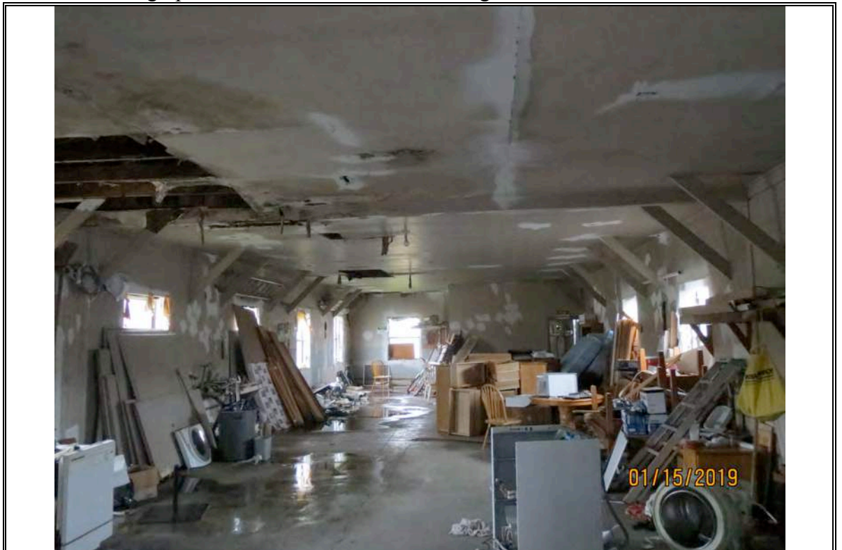
Photograph Number 10: View of the building interior
