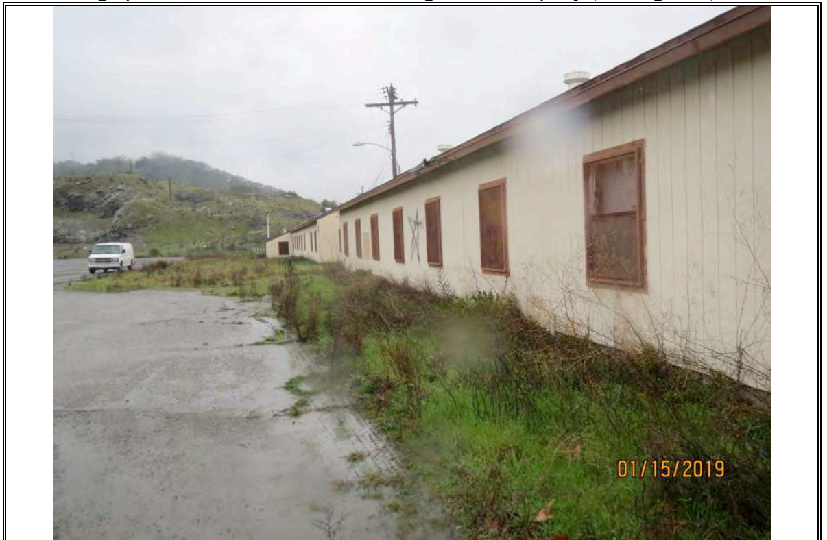
Photograph Number 4: View of the buildings on the Property (looking west)
