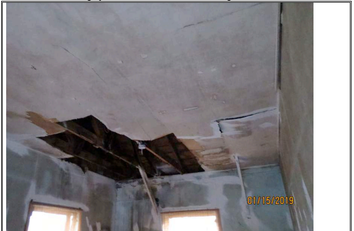
Photograph Number 8: View of the building interior
