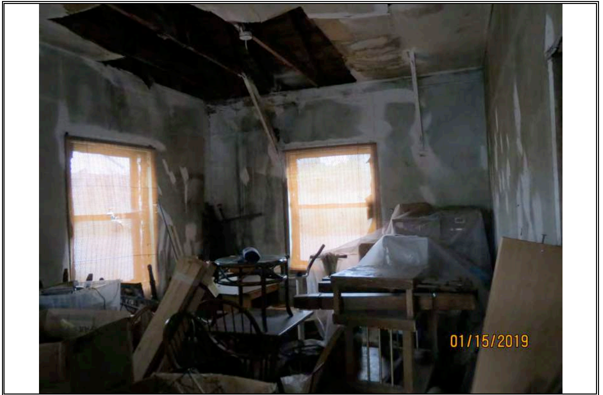
Photograph Number 7: View of the building interior
