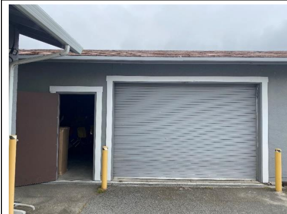
Photo 15: View of Workshop building located behind 100 Commodore Webster Drive.
