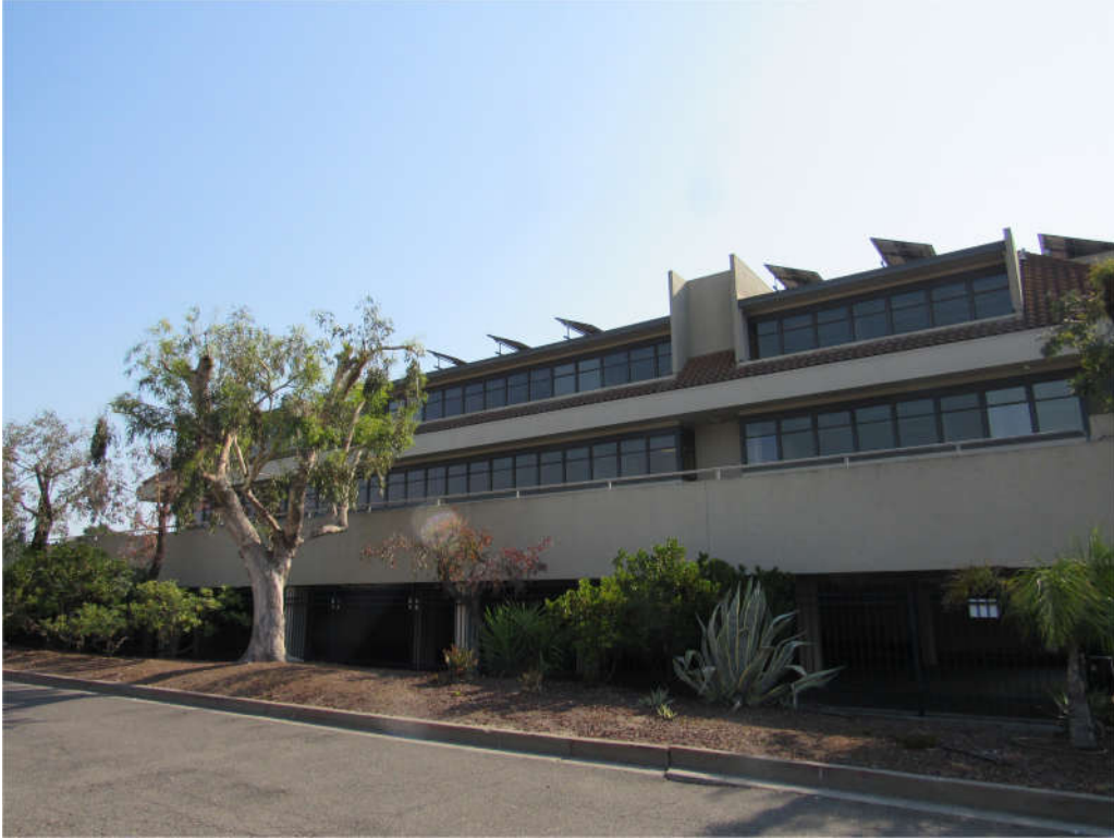
Rear view of the building
