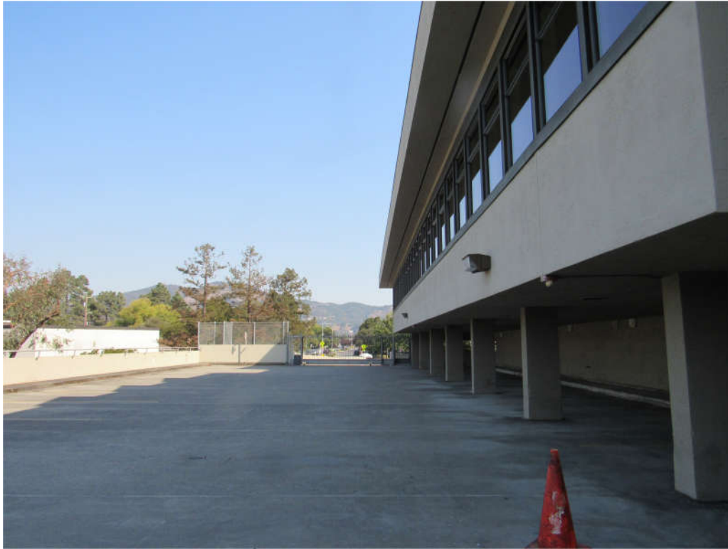
Parking garage – 2 nd level open parking- ramp from Kerner Blvd.
