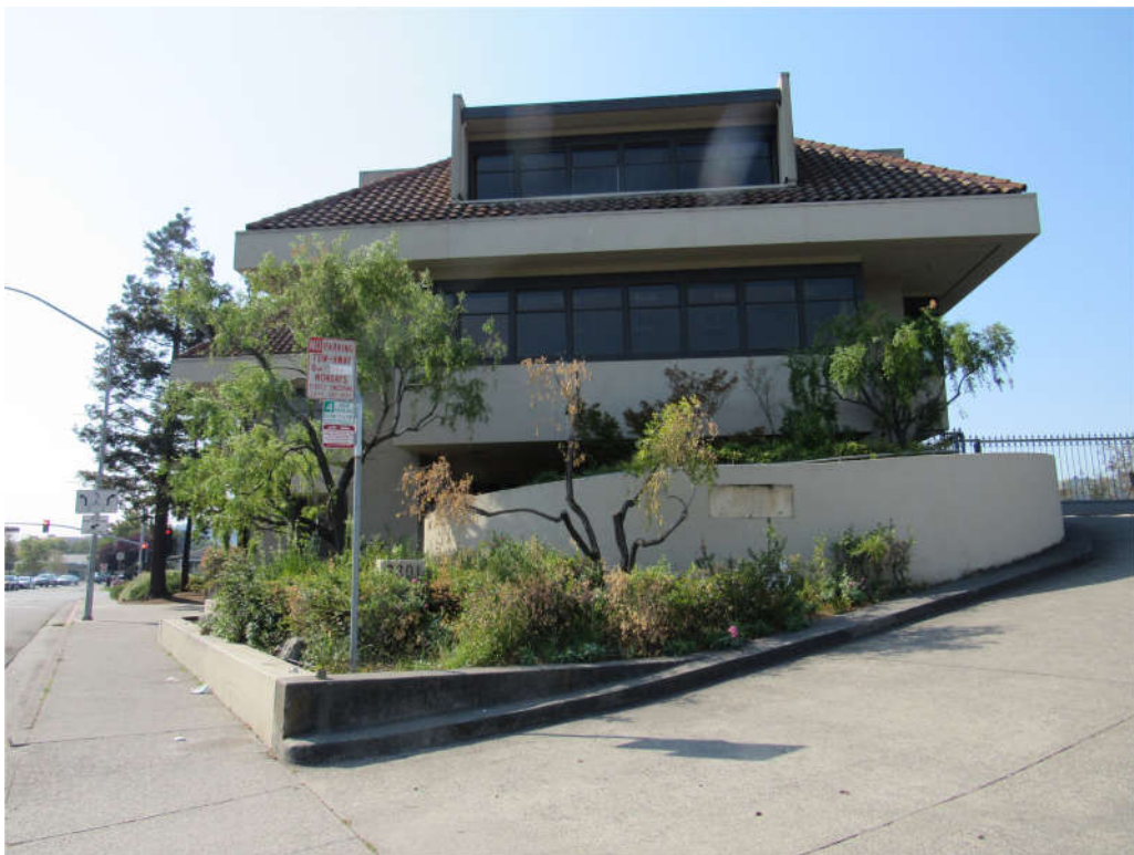
Northeast side of building
