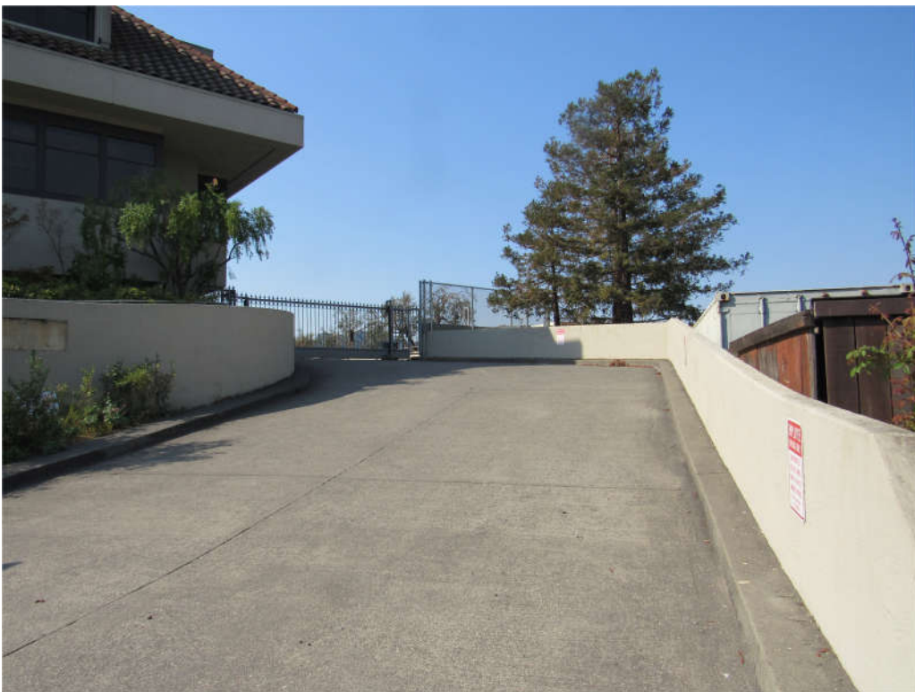
Ramp from Kerner Boulevard to parking area
