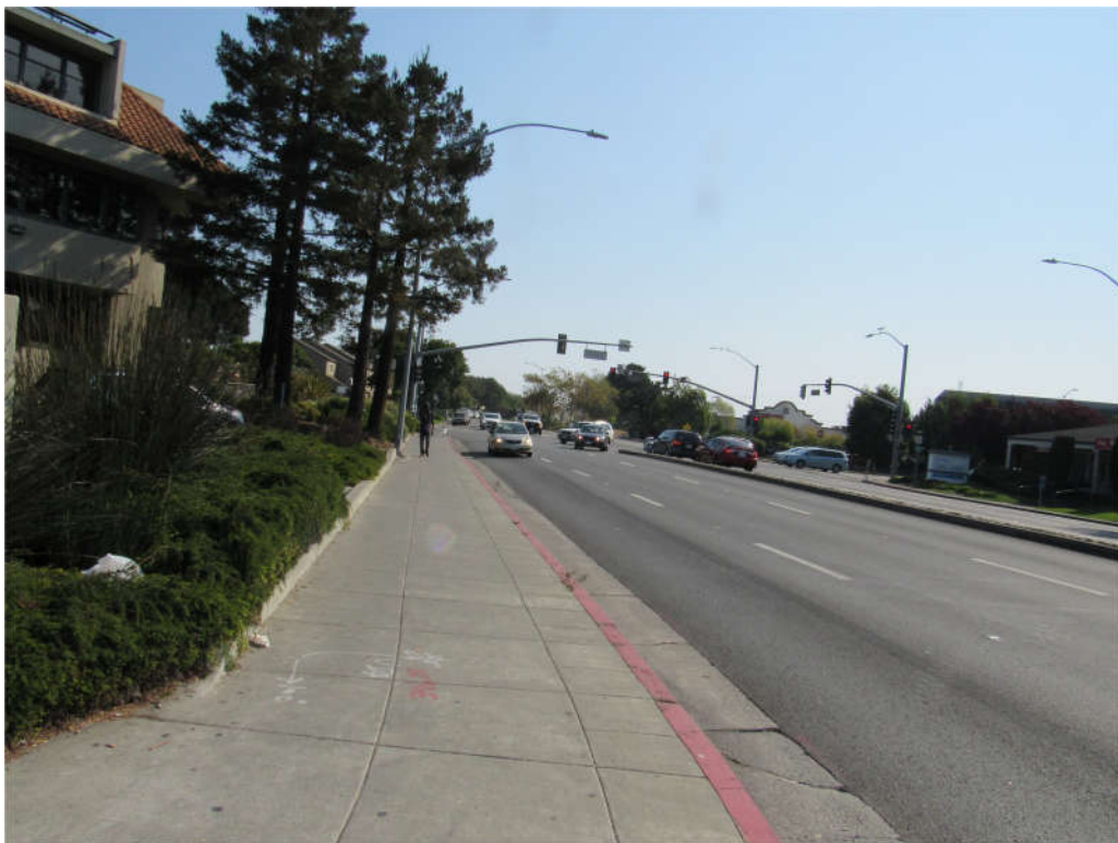
View northeast on Bellam Boulevard
