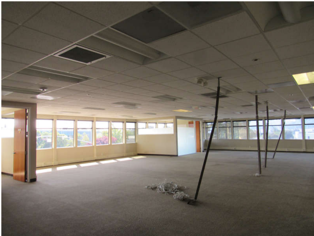
2 nd floor office – with some private offices built-in
