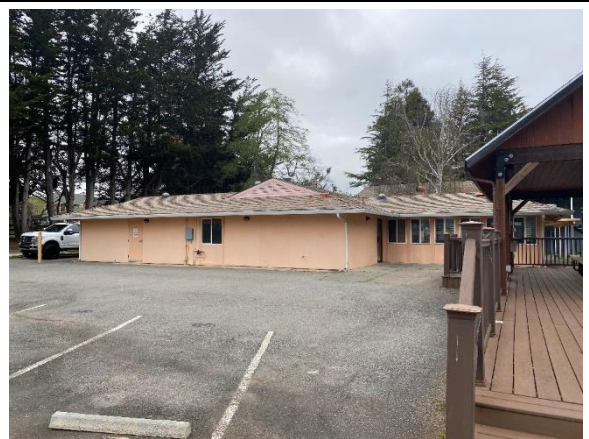
Photo 6: View of Galley Building.
