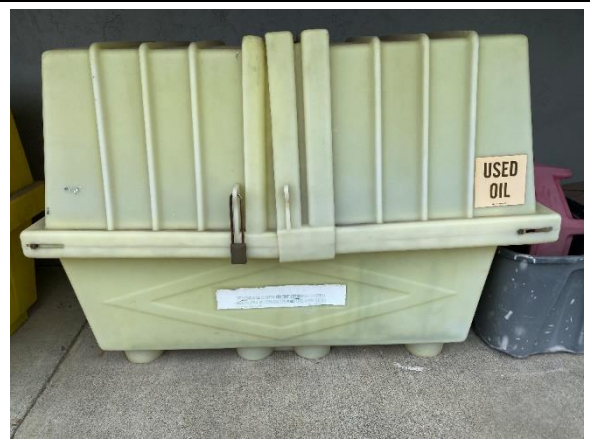
Photo 21: View of used oil secondary containment located behind the Workshop Building.
