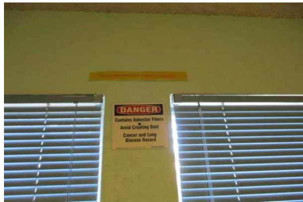
#64: INTERIOR CEILING FINISH, GYPSUM BOARD/PLASTER
