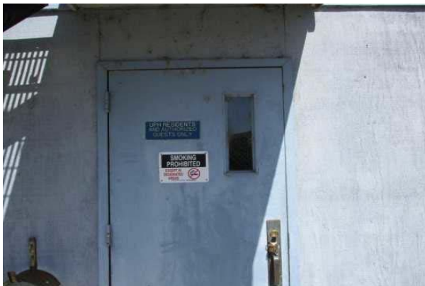
#41: EXTERIOR DOOR, STEEL WITH SAFETY GLASS
