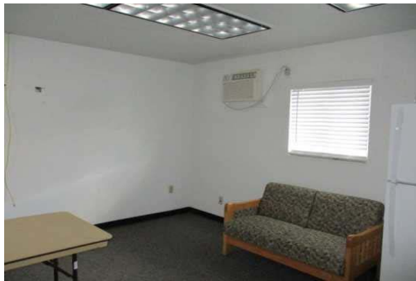
#63: INTERIOR WALL FINISH, GENERAL SURFACE
