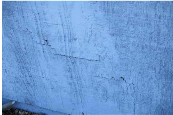
#38: EXTERIOR WALL, BUILDING 50
