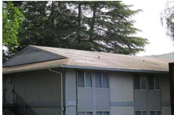
#34: BUILDING 50 ASPHALT SHINGLE
