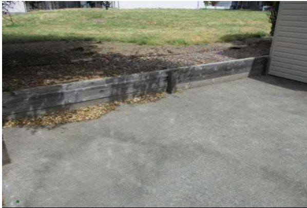
#31: RETAINING WALL, TREATED TIMBER
