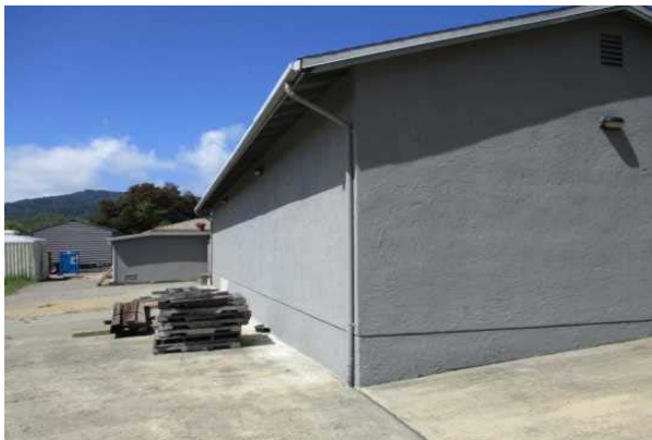
#11: REAR OF THE STORAGE BUILDING
