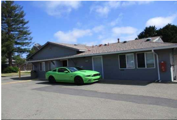
#1: FRONT OF BUILDING 100
