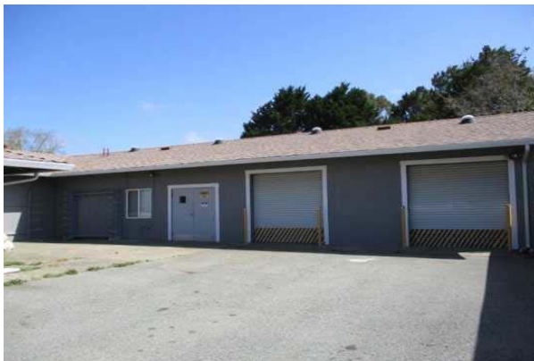
#35: BUILDING 100 ASPHALT SHINGLE
