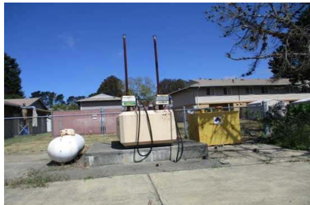
#54: FUEL STORAGE TANKS
