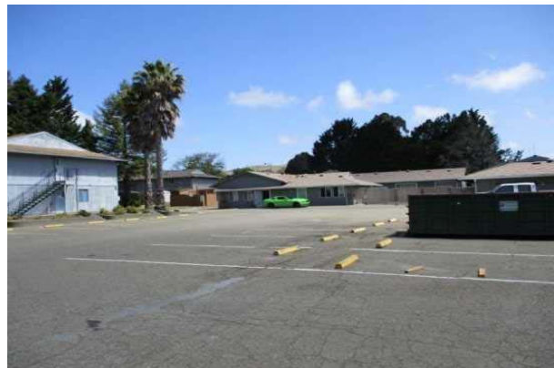
#30: PARKING LOTS, ASPHALT PAVEMENT
