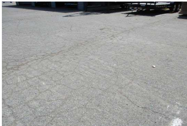
#29: PARKING LOTS, ASPHALT PAVEMENT
