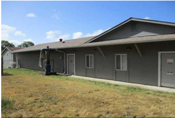
#37: EXTERIOR WALL, PAINTED SURFACE
