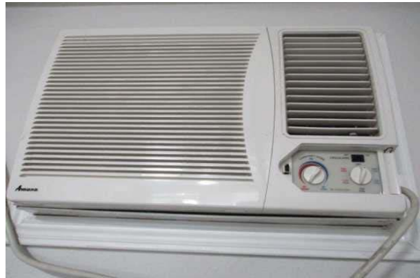
#46: PACKAGED TERMINAL AIR CONDITIONER (PTAC)
