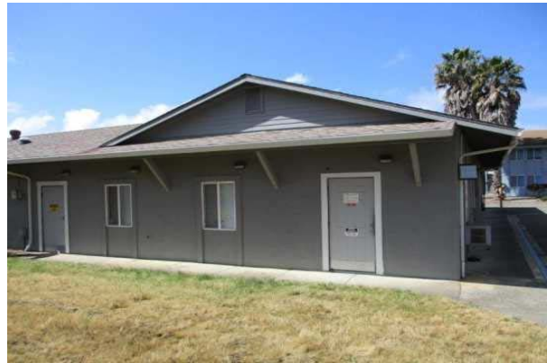
#4: REAR OF BUILDING 100
