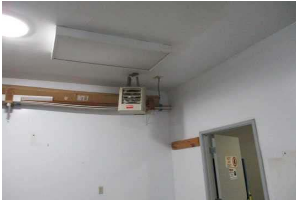
#45: UNIT HEATER, ELECTRIC
