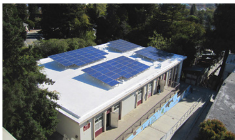
Roof mounted solar - Santa Cruz USD
