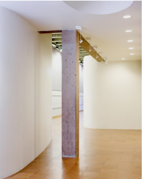
Hallway with existing column
