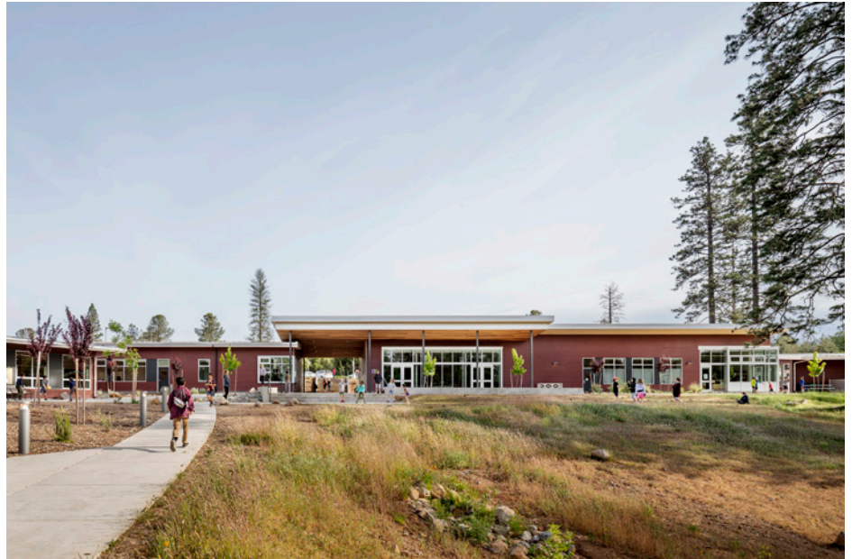
View up the hill toward multipurpose room, library & administration wing
