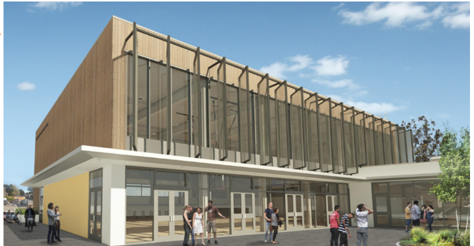
Bushnell Center view from courtyard highlighting fog catchment "sails."
