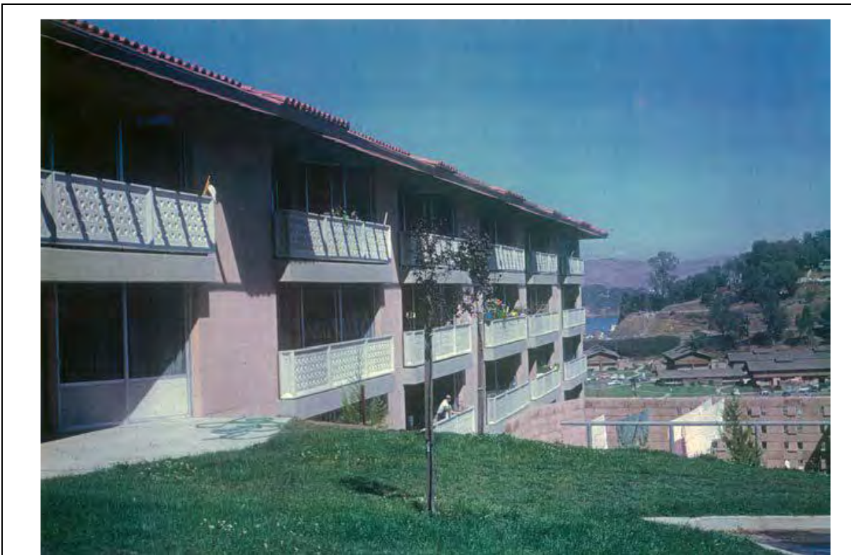
Figure 27. The historic condition of the façade at the rear of the high-rise buildings in 1961, illustrating the precast balcony guardrails with the exposed rafters overhead and the warm clay/pink color of the concrete façade. Source: Ruark, 2017.
