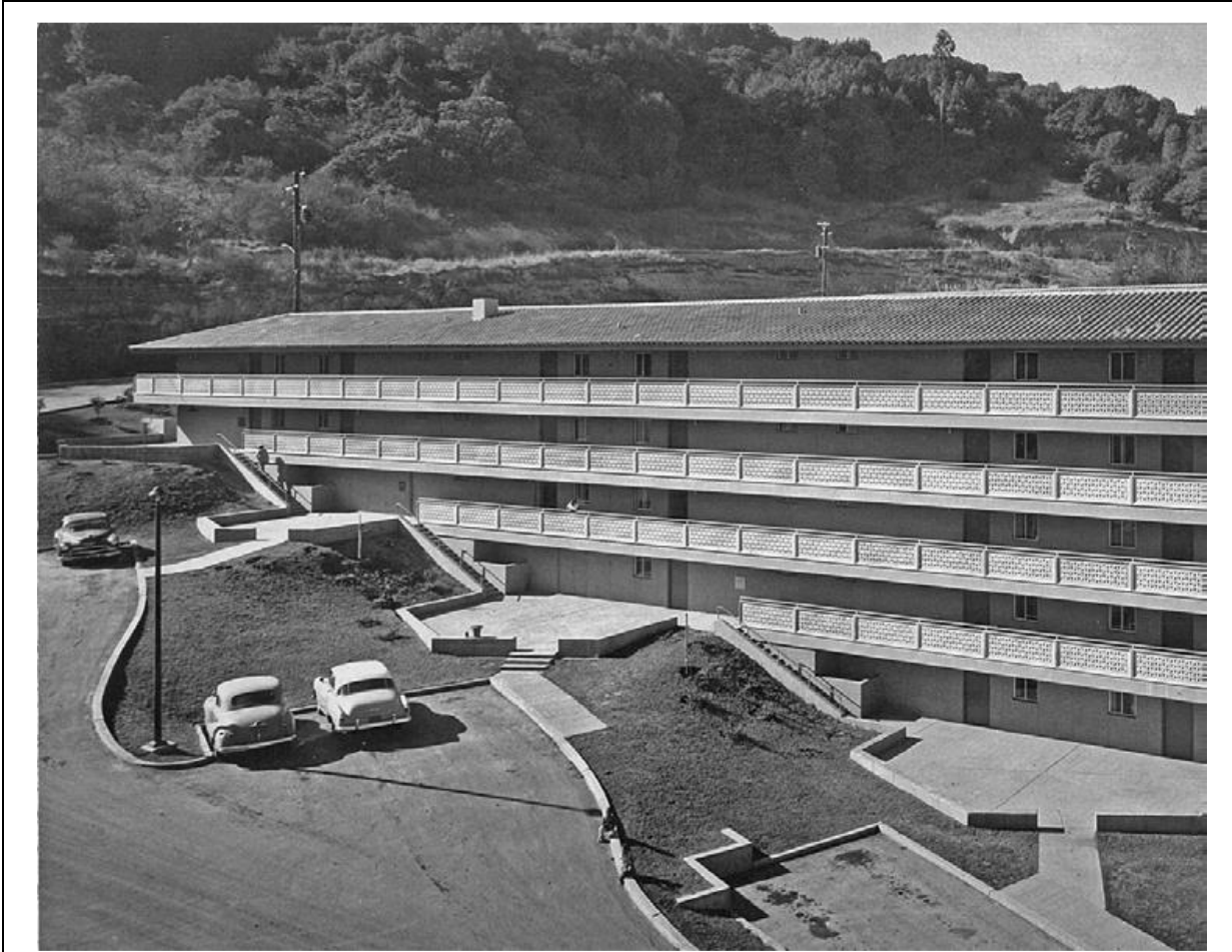
Figure 26. The historic condition of the precast concrete guardrails along the front façade of the high-rises, ca. 1961. Source: Ruark, 2017.
