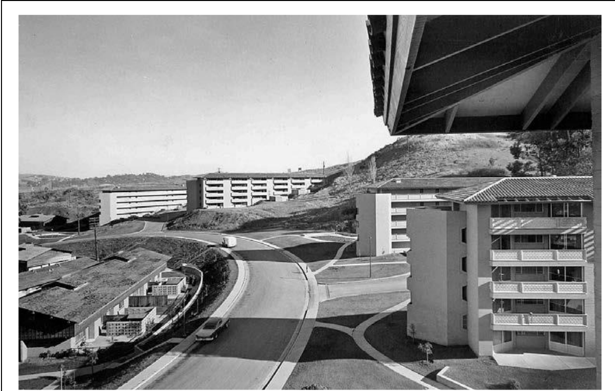
Figure 25. The historic condition of the enclosed stairwells at 69 and 79 Cole Drive, ca 1961. Source: Ruark, 2017.
