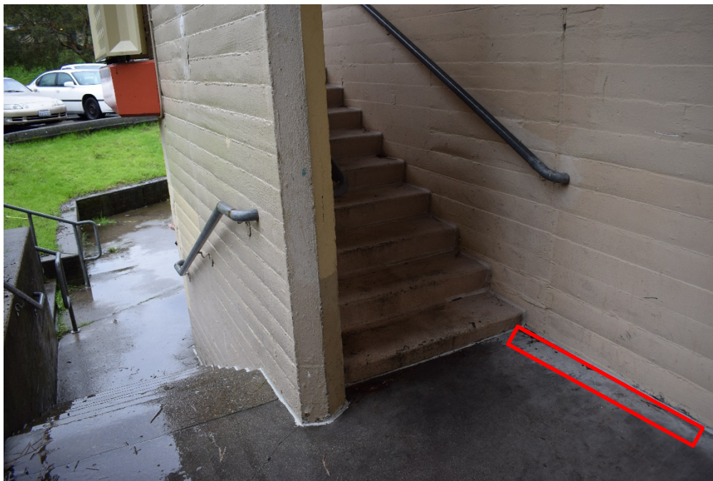
Figure 5: Photograph of the proposed French drain location (outlined in red), which would run under the existing stairway and up to the ground level landing, and continue east along the building's south façade, roughly within the area outlined in red. Courtesy: ICF 2020.
