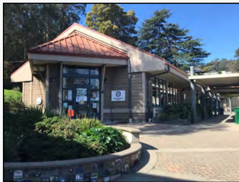
WILLOW CREEK ACADEMY 630 NEVADA STREET SAUSALITO, CALIFORNIA 94965
