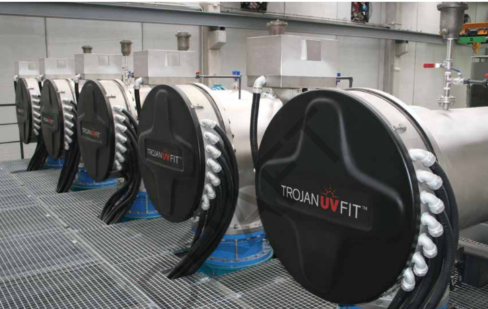
WASTEWATER DISINFECTION FILTERED IN-PIPE TREATMENT
