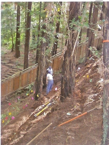
A steep slope installation in California — 65% slope.
