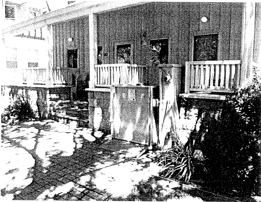
Entry porch at 82 Park (Community Building)
