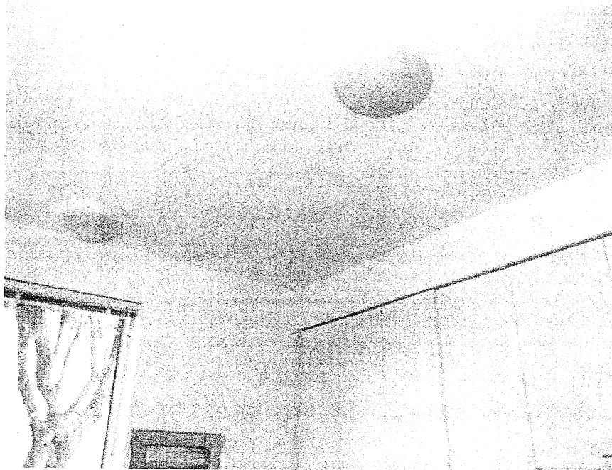
Typical ceiling fixtures at kitchen
