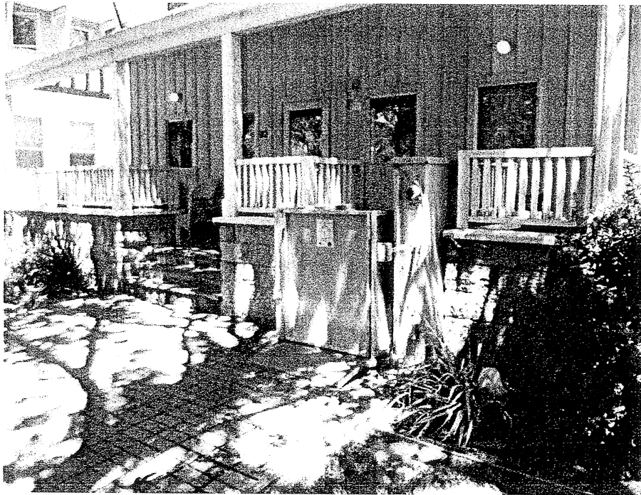
Entry porch at 82 Park (Community Building)
