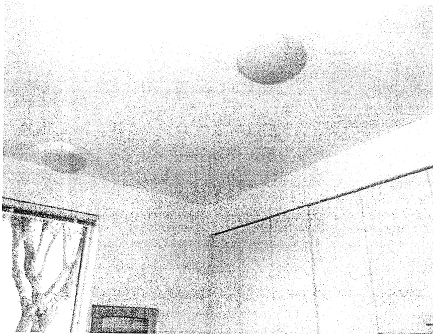
Typical ceiling fixtures at kitchen
