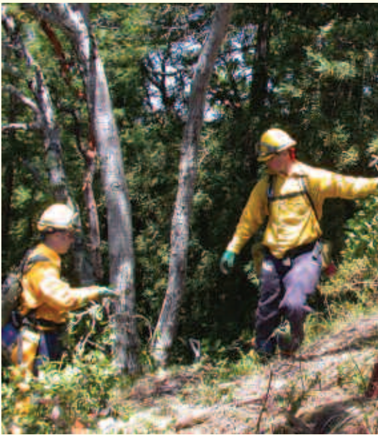
Clearing vegetation along Indian Fire Road
